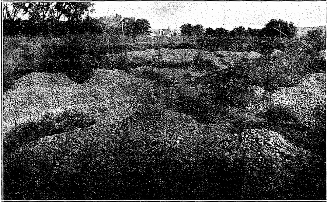
Figure 13. Pit Showing Waste of "Oversize"
