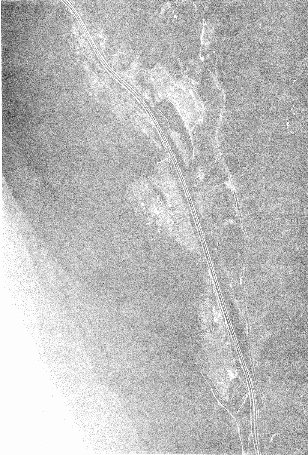
Figure 16. Interstate 26 Slide Area, May, 1977.
