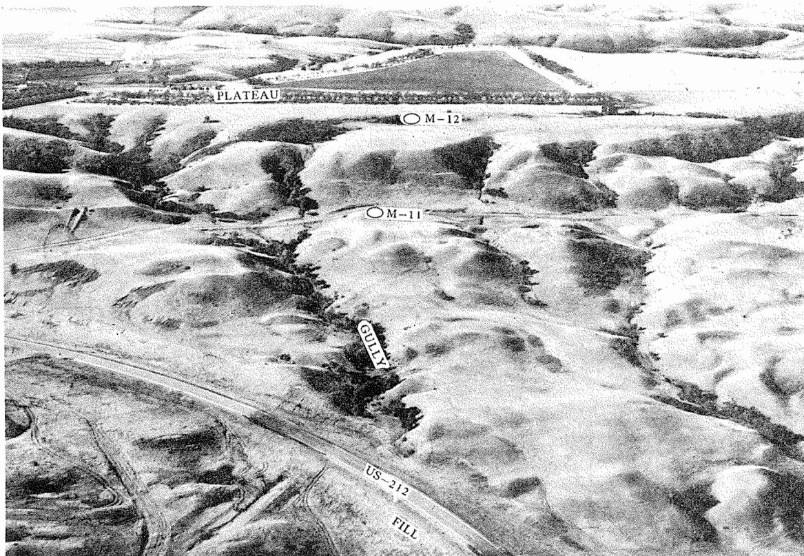
Figure 4. Oblique photograph of back scarp area, looking south, 1962.
