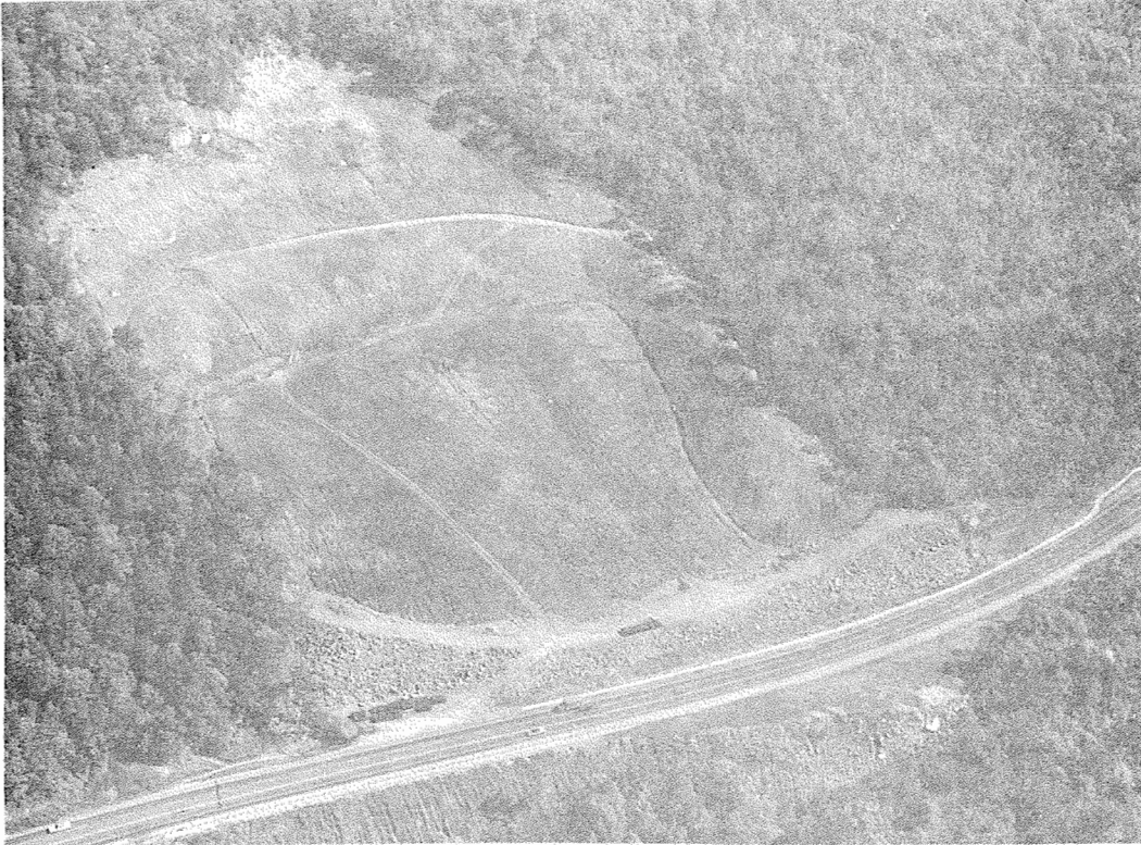
Figure 23. Aerial View of Repaired Slide #8 Along I-40 at Rockwood (see Figure 22).
