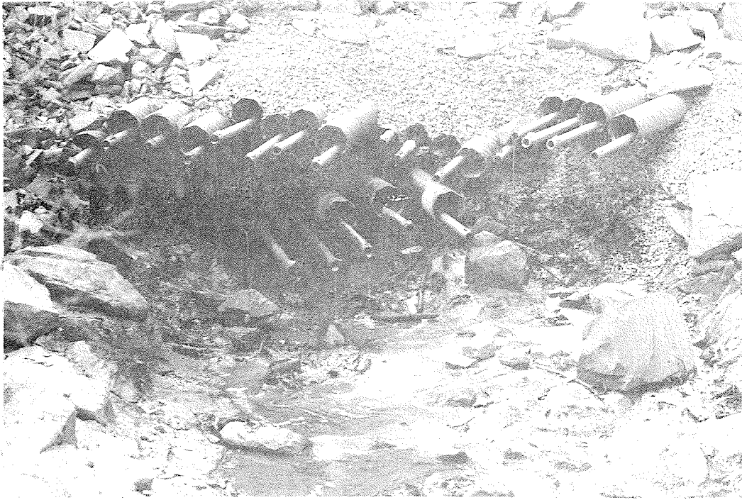
Figure 26. Horizontal Drain Installation at Rockwood (see Pad "B", Figure 25).
