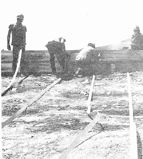
Photo 6. Attaching reinforcing elements to 13 inch face "skins".
