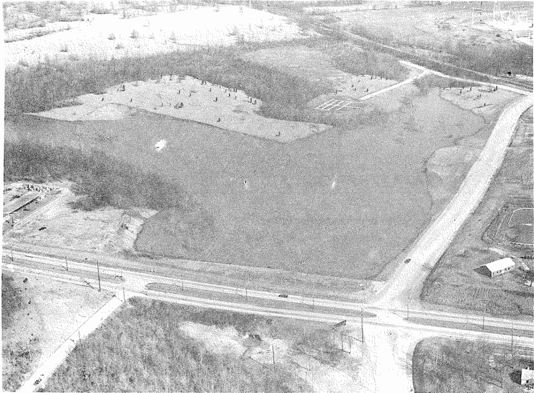
Figure 5. Aerial View of State Route #1 Horizontal Drain Project. (Note outlet end of Box Culvert in lower part of photo.)
