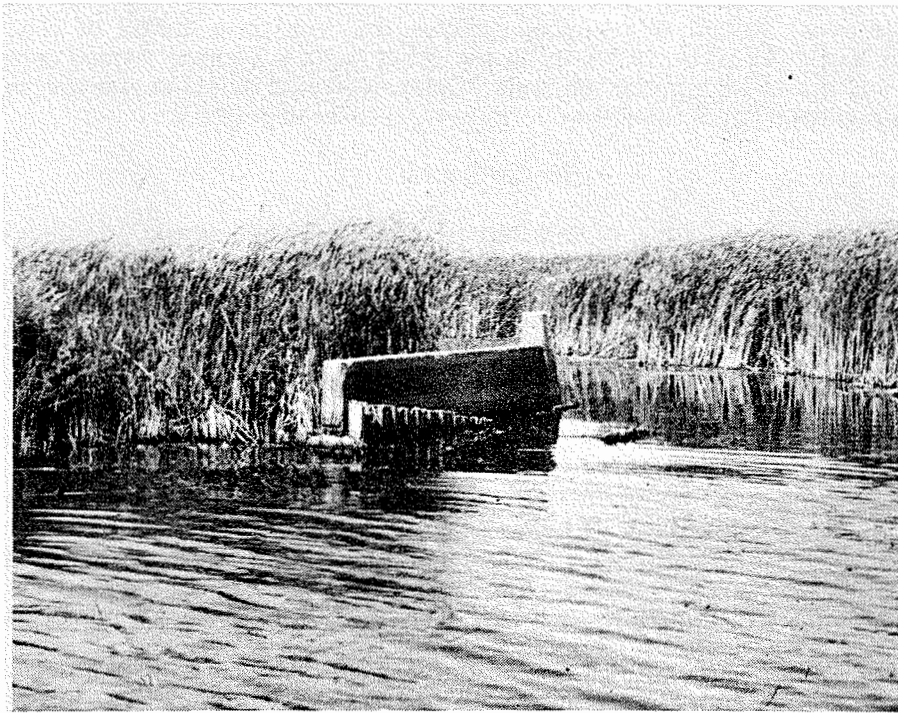
Figure 4. Photograph showing the remains of a concrete weir constructed in 1928.
