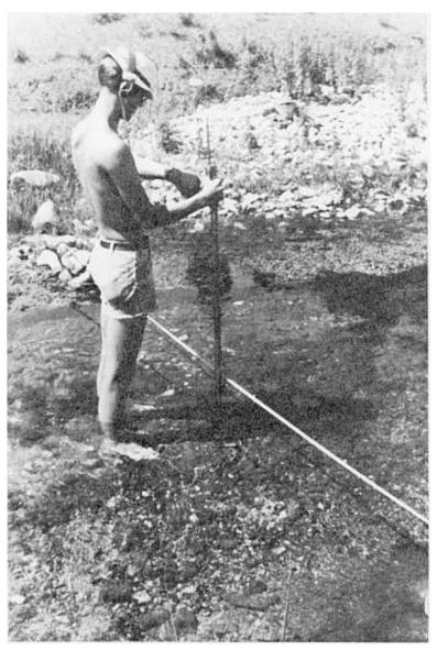
Figure 2. Beaver Creek at Buffalo Gap (Site 15) is being gaged with the pigmy current meter. Twenty readings of the average velocity, as determined by a spinning wheel in the current, is multiplied by the cross-sectional area to determine the total discharge.
