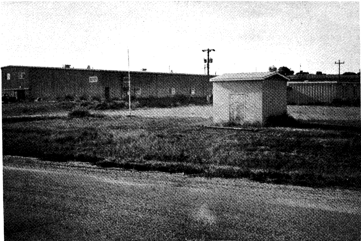
Figure 2. Photograph of the municipal well at Midland, S. D. The small building in the foreground houses the Midland city well. Hot water from this well heats the gymnasium in left background and the classroom building in right background.
