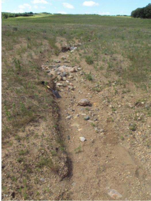
Figure 19. Small gully forming on mine floor.
