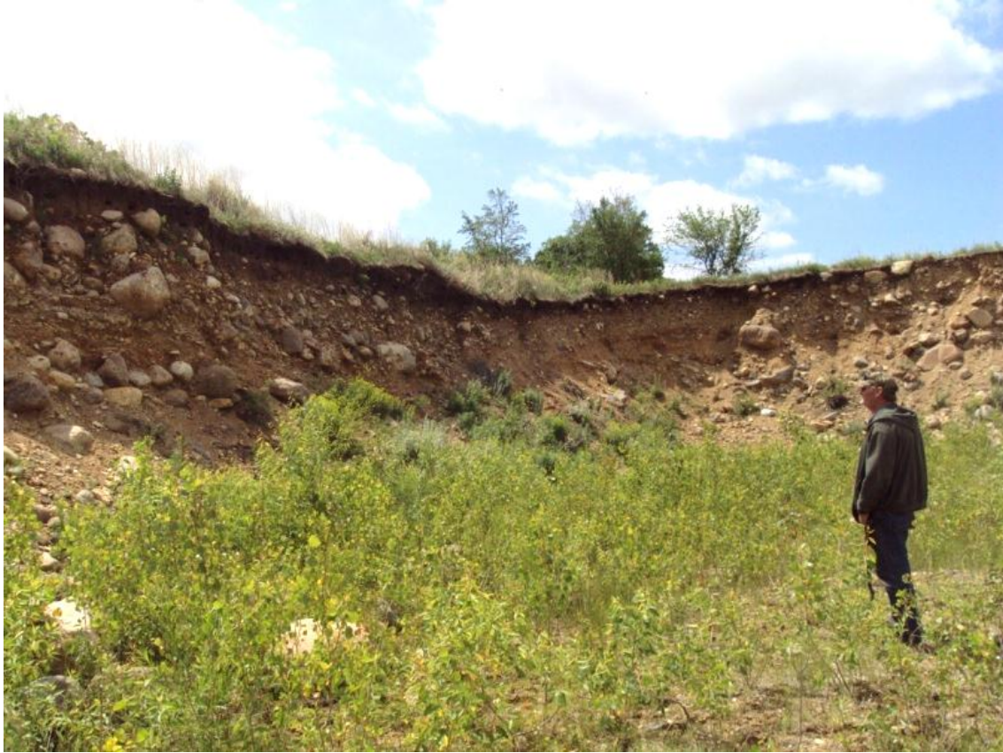
Figure 4. View of the mine wall in the northwestern area.
